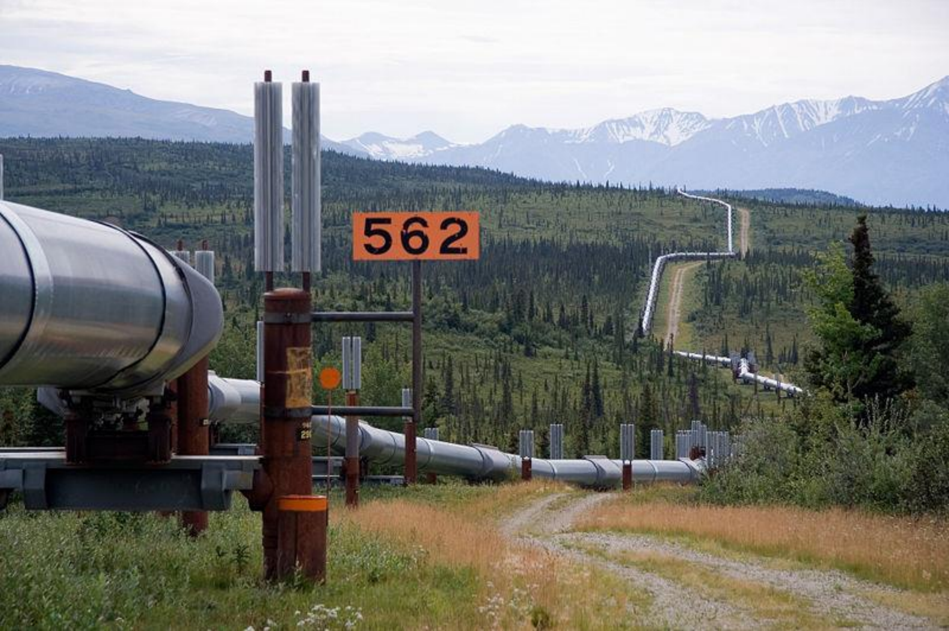
Trans-Alaska Pipeline System
