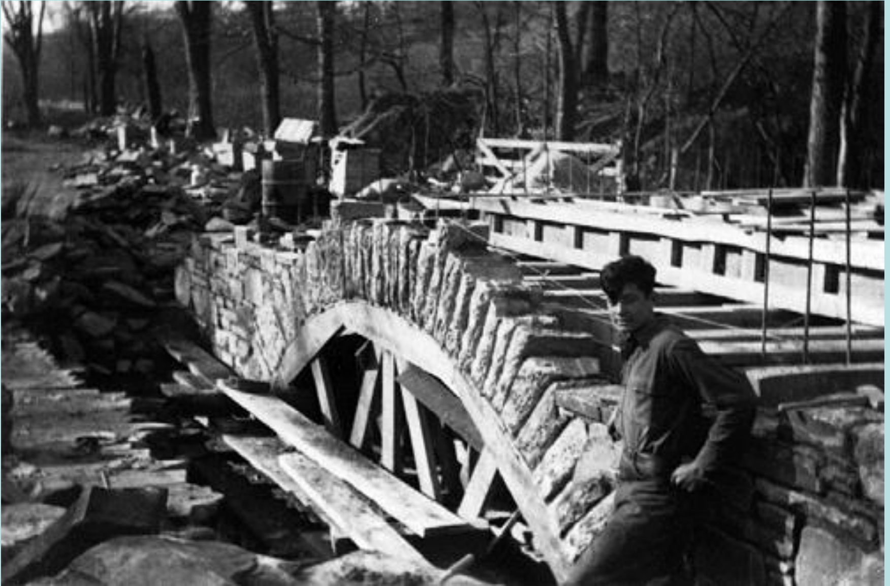
Worker During Bridge Construction, Staatsburg, NY
