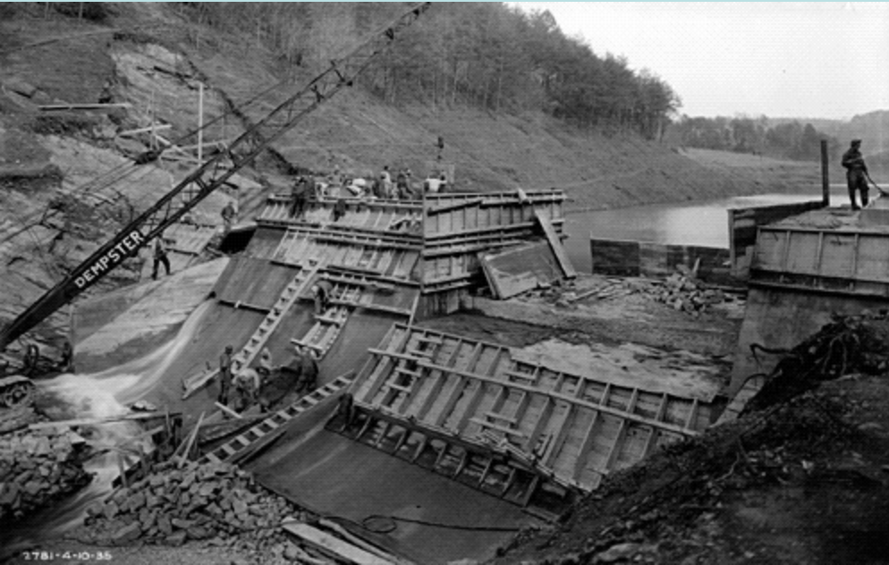
Building Big Ridge Dam (TN)
