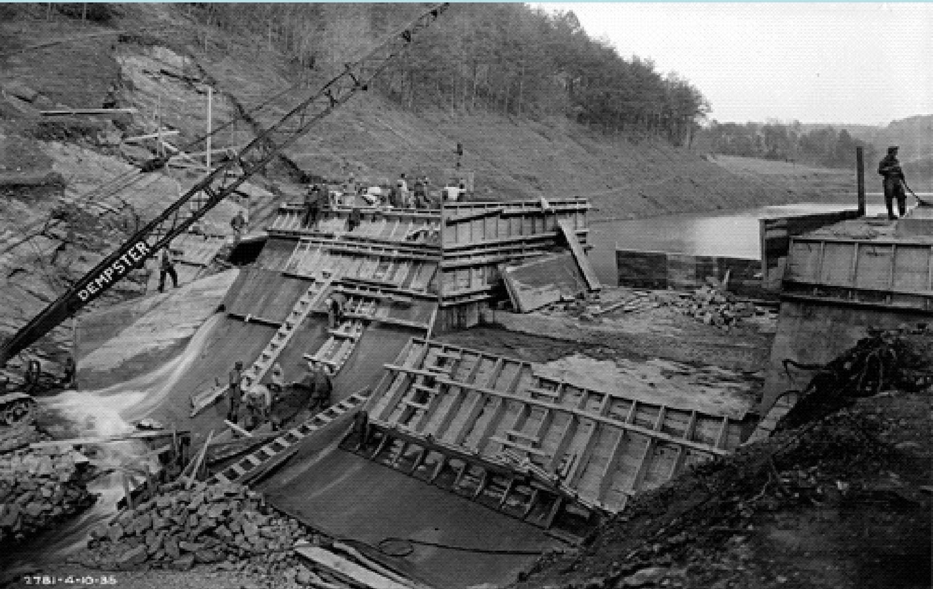
Building Big Ridge Dam (TN)
