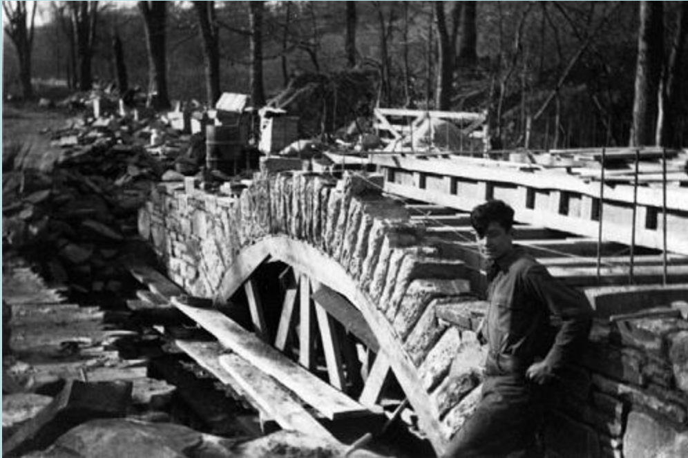
Worker During Bridge Construction Staatsburg, NY
