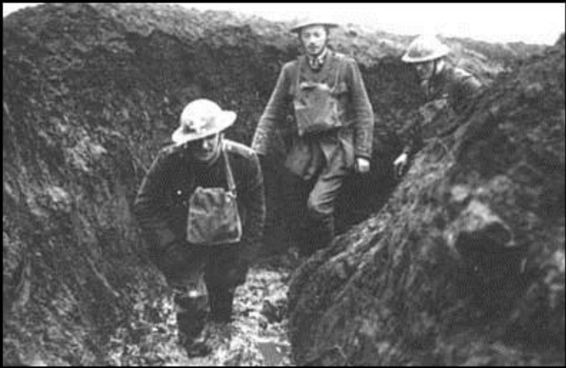
Officers walking through a flooded communication trench.
