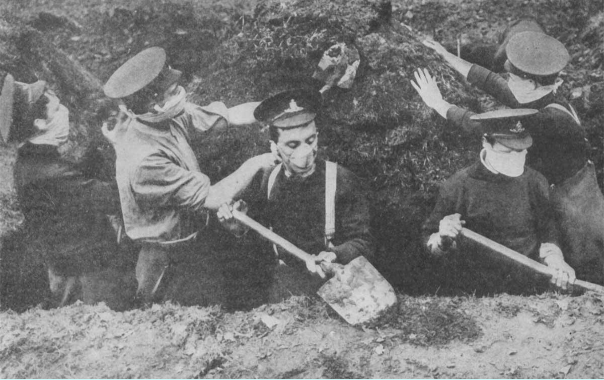
Soldiers digging trenches while protected against gas attacks
