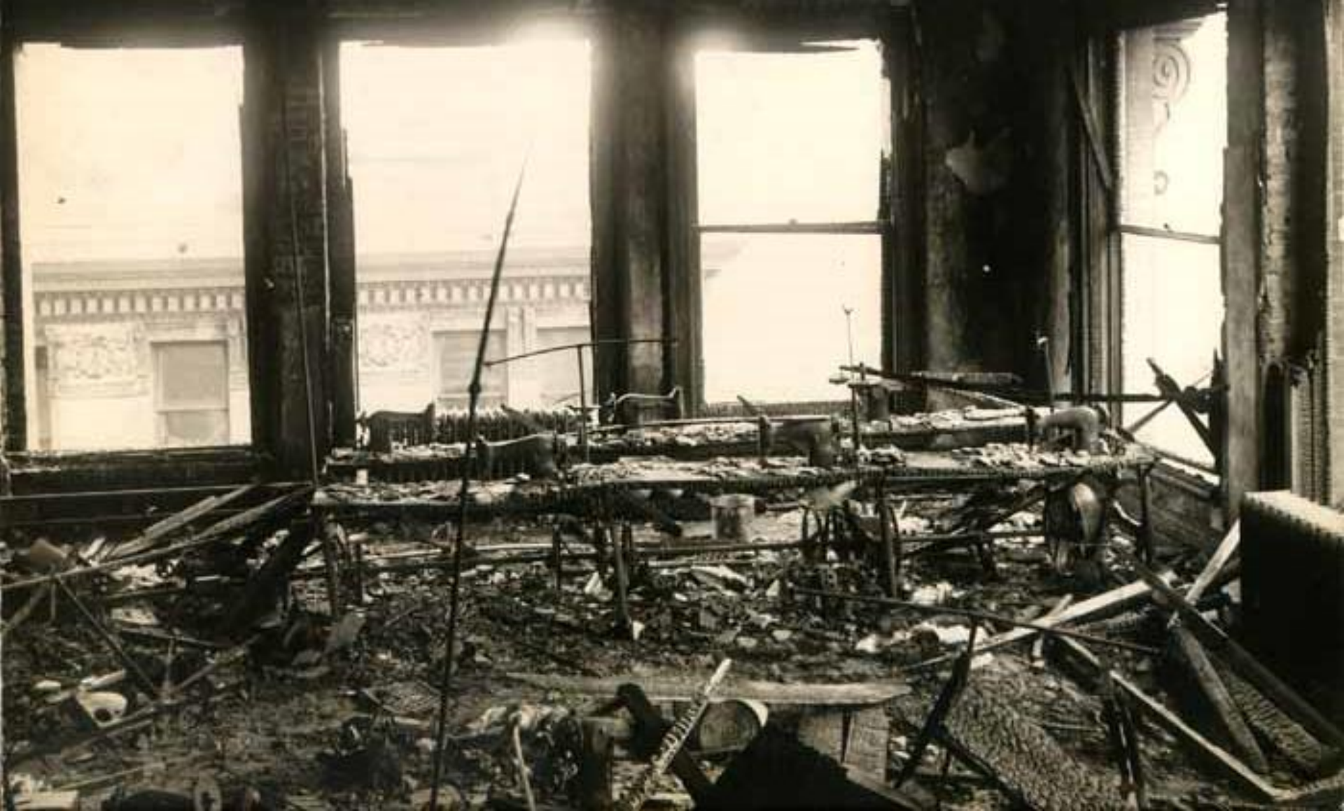
The 240 employees sewing shirtwaists on the ninth floor had their escape blocked by back-to-back chairs and workbaskets in the aisles. The 75-foot long paired sewing machine tables obstructed essential access to the windows, stairs, and elevators.
