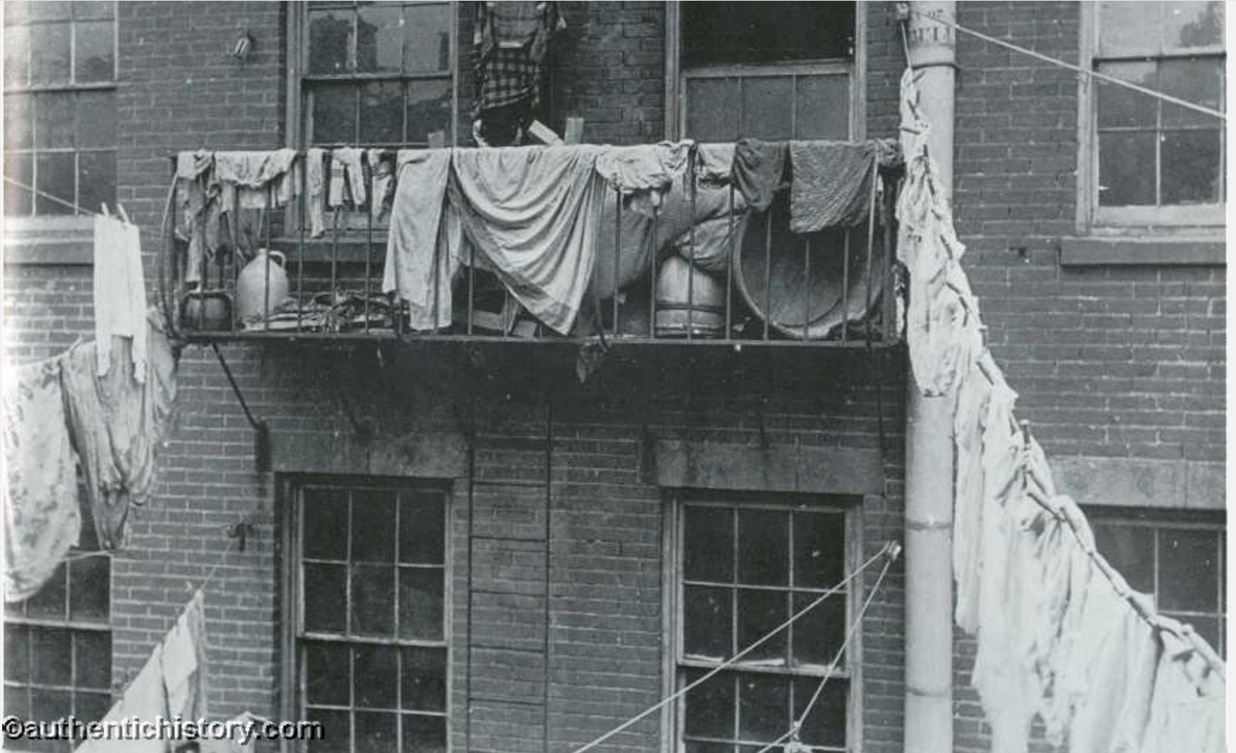
Typical tenement fire-escape serving as an extension of the flat: Allen Street
